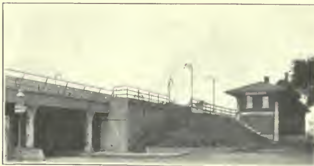
FIG. 308. SUBURBAN STATIONS. Station at Rogers Park, Chicago & North Western Railway.
